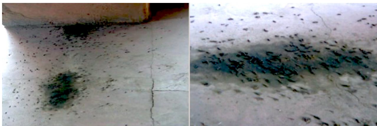
Figure 4. Accumulation of Bat Guano in Interior Spaces of Chander Nagar Gate, Lucknow.
