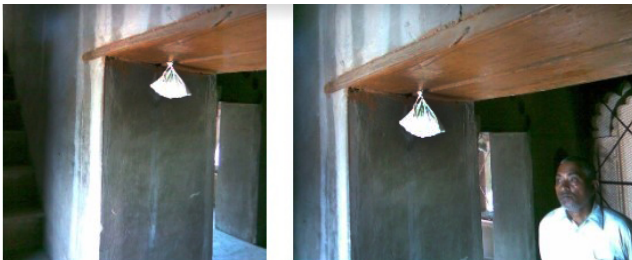
Figure 5. Use of Naphthalene Bags as A Chemical Deterrent in the Interior of Chander Nagar Gate, Lucknow.
